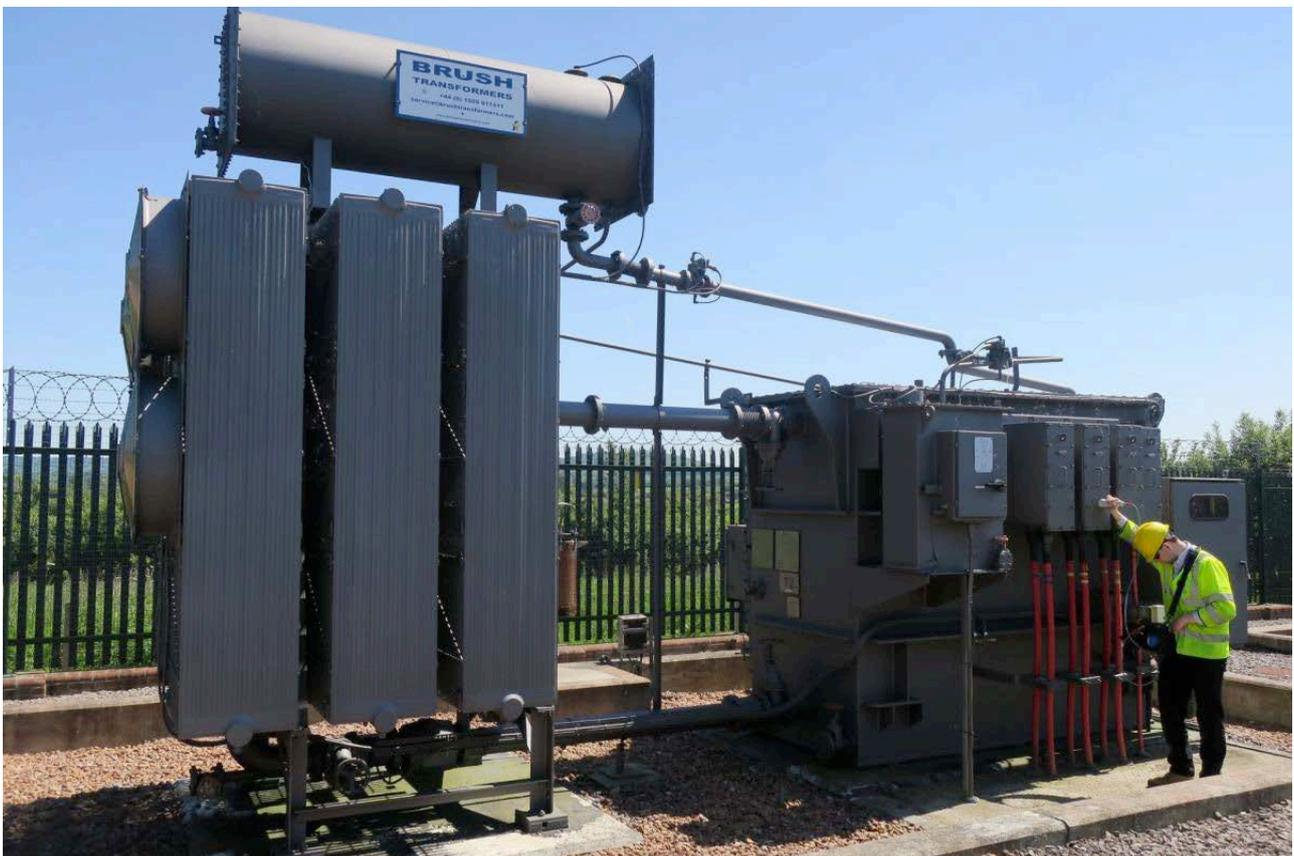
Figure 4-9 - SSEN 15MVA transformer
