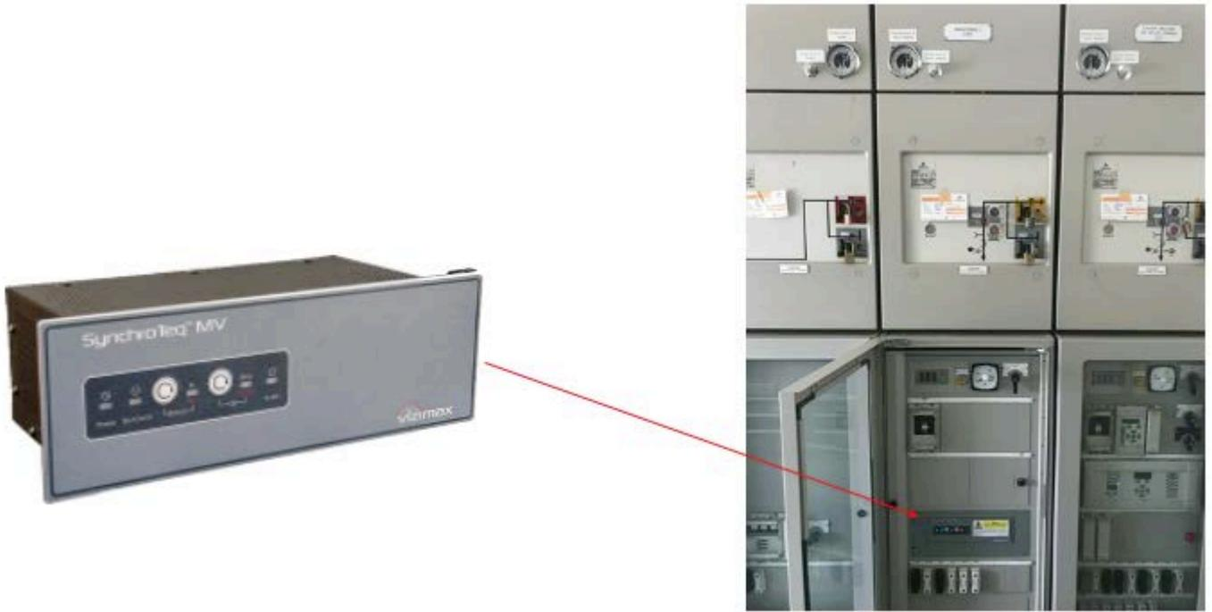
Figure 4-10 - SynchroTeq Installed within Switchgear
