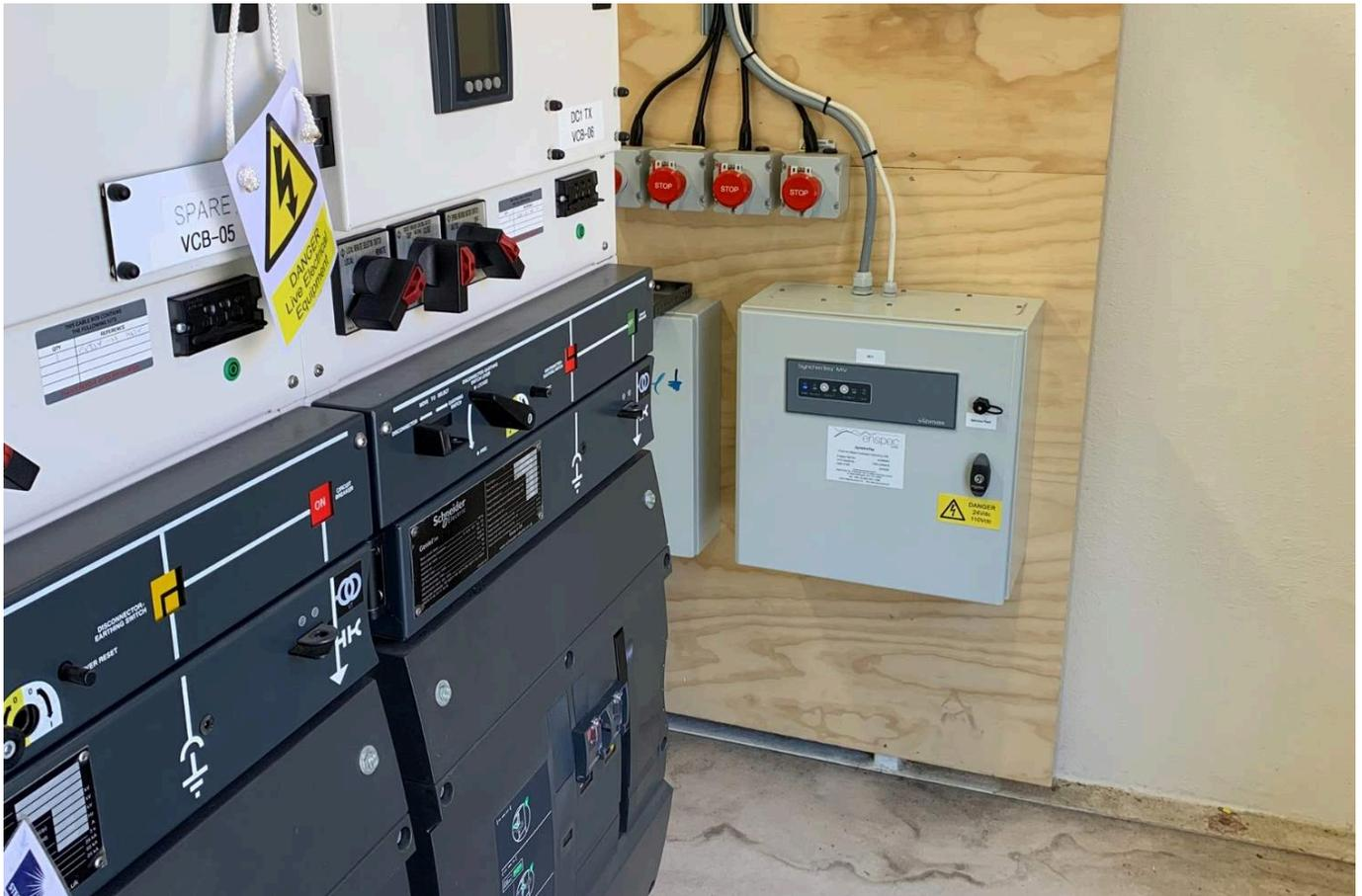
Figure 4-6 - SynchroTeq Retrofit Installation
